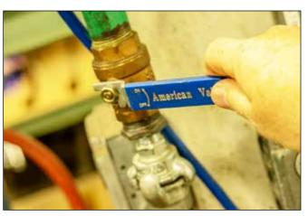
**6.** Turn compressed air supply **ON**. Inspect compressed air hose for air leaks
