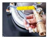
4. Install the 1/4" OD tubing into both push-to-connect elbows. Ensure the tubing is fully seated in the fitting. A slightly added resistance will be felt before the tube is fully seated. Once fully seated, test the connection by firmly pulling on the tube. It should stay locked in the fitting.
