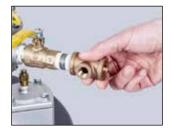
2. Install the ½" to ¼" pipe tee reducer onto the pipe nipple. Orientate the ¼" outlet of the pipe tee to the same side of the manifold with the ¼" push-to-connect elbow installed.
